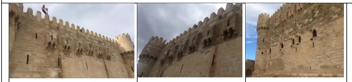
Fig. (13) The northern and western facade of the tower of the citadel.
